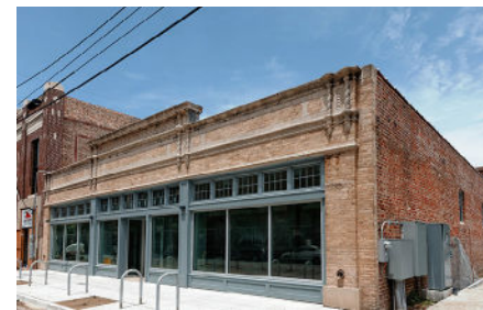
Photo credits: FH Myers Construction
